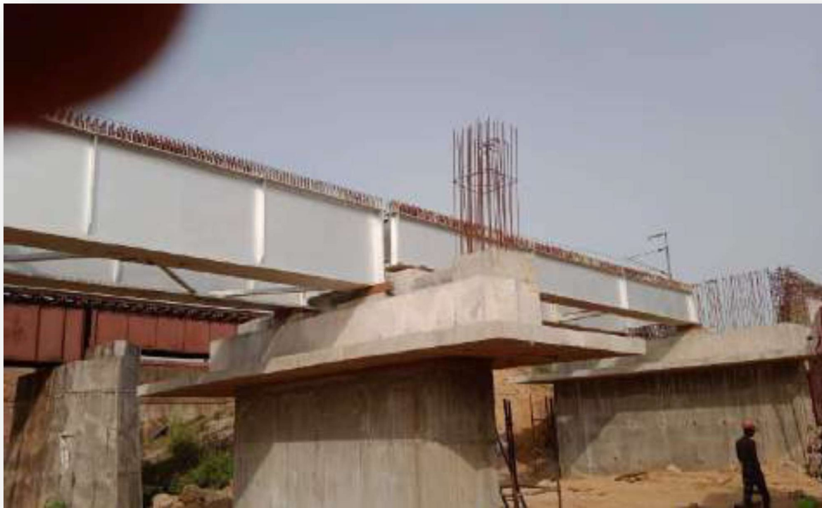
18.3x2 Span & 12.2x2 Span Fabrication & Erection @ 192 Nos Bridge Sisigi Jharkhand (RVNL PKG -2 Japla
