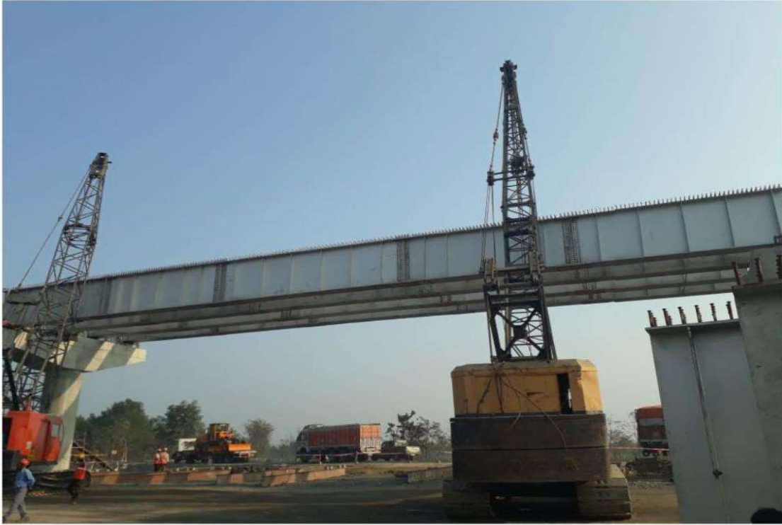
39 M SPAN GIRDER
