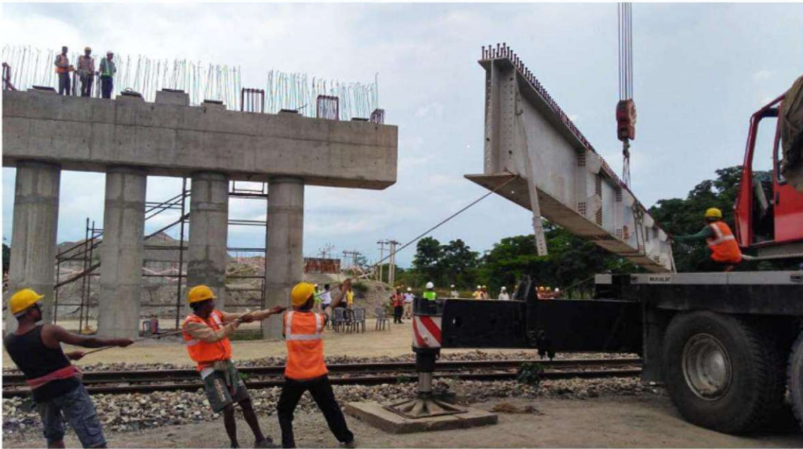
24 M SPANRDSO ROB GIRDERS LAUNCHING
