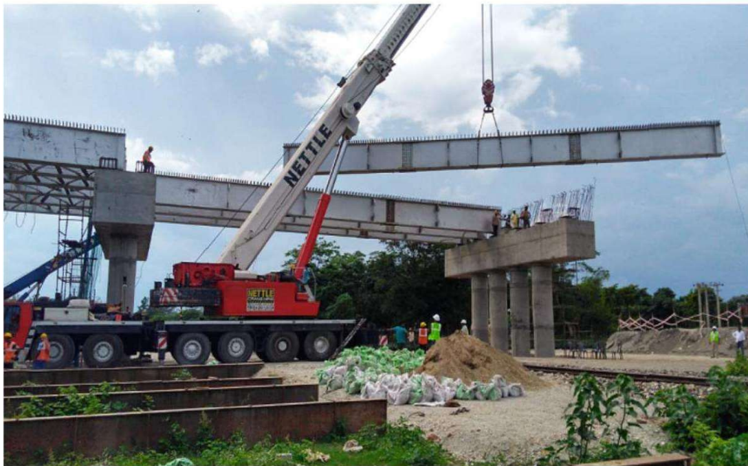
24 M SPANRDSO ROB GIRDERS LAUNCHING
