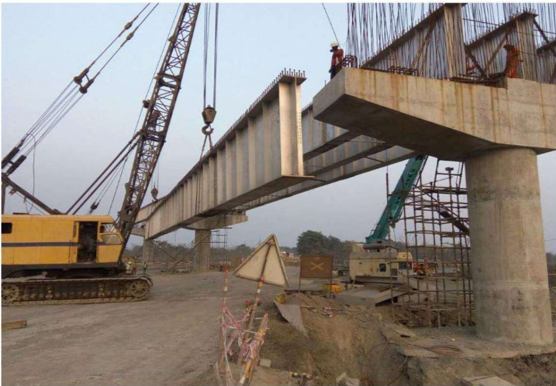
39 M SPAN GIRDER
